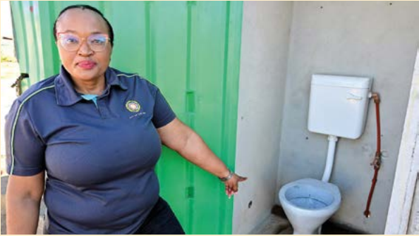
Dignified sanitation: City technician Nosithandiwe Mene at one of the newly installed full-flush toilets in Overcome Heights.
